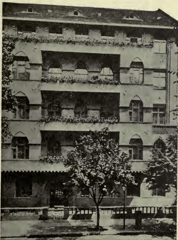
FROM "THE CRAFTSMAN" BERLIN APARTMENT-HOUSE WITH CONCRETE TROUGHS FOR BALCONY FLOWER GARDENS
